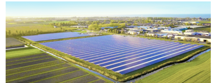
Buinerveen 41MW Solar Power Plant
