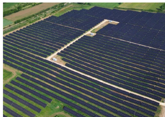
Saraorci 13.86MWp PVPP Project
