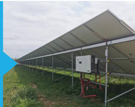
6MW Ground PV EPC Project
