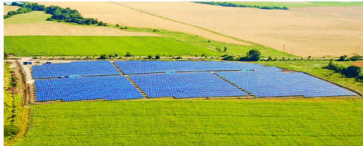
Bezmer 10MW Solar Power Plant
