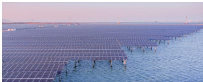
Wenzhou 550MW Fishery-Solar Complementary Power Station
