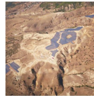
Aydin 10.7MW Solar Power Plant
