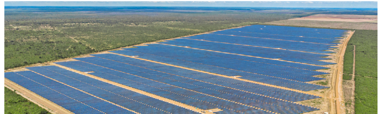
Barreiras 50MW Solar Power Station
