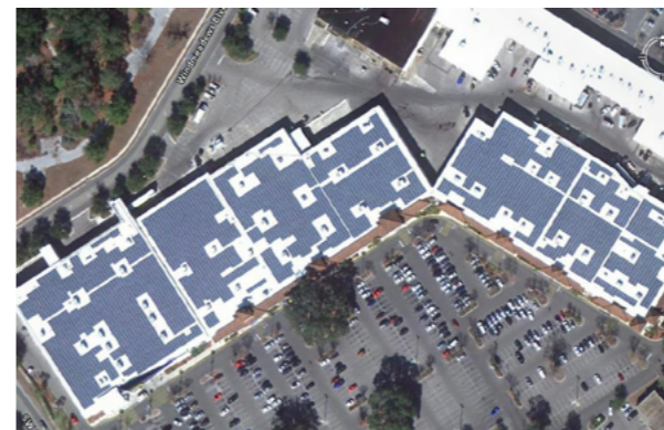
Gainesville Butler Plaza 2.2MW Solar Power Plant
