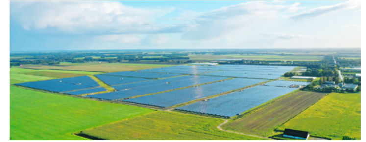
Veendam 15.5MW Solar Power Plant
