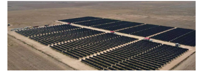
1074 Copper Coast Highway 5.9MW Ground Solar Power Plant
