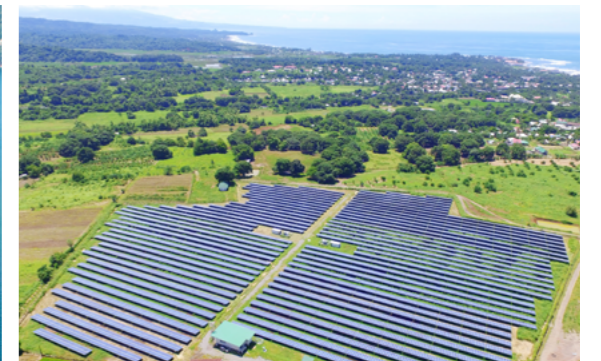
THE PHILIPPINES | Bataan 5MW Solar Power Plant
