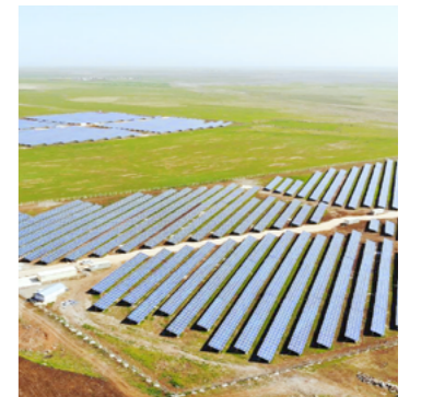
URFA 13.82MW Solar Power Plant
