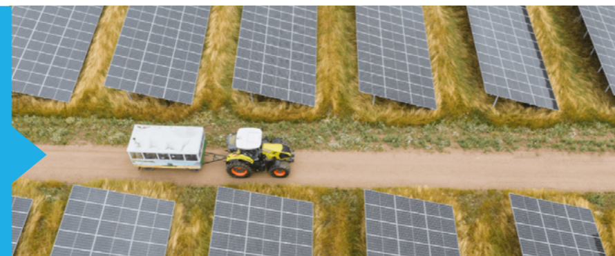
Brandenburg Döllen 154.4MW Solar Power Plant
