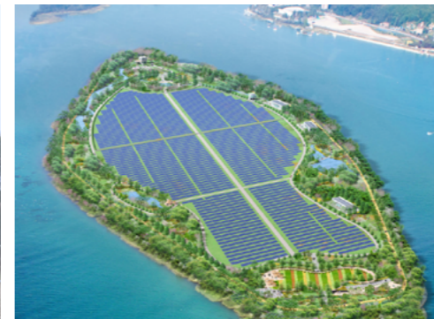
KOREA | Boongeo 9MW Solar Power Plant
