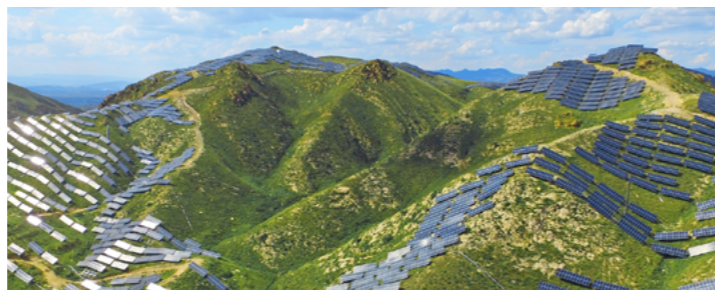
Zhangjiakou 70MW Solar Power Station
