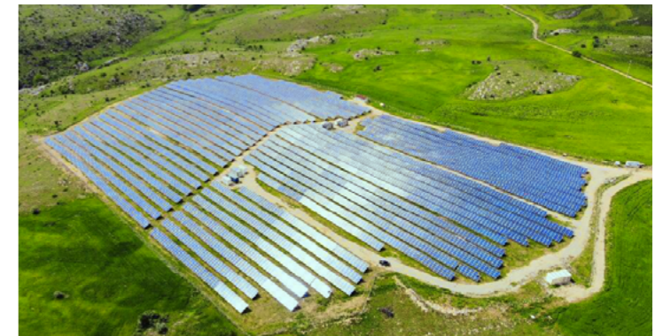
Elmadag 4.78MW Solar Power Plant
