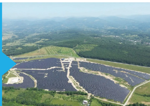
CEF Slătioara 31.6MW PV Power Station
