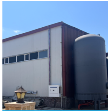
Winery 450kW Rooftop Project
