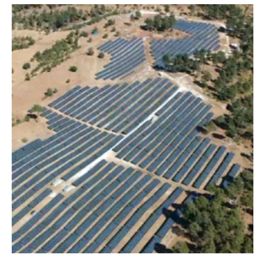
Maras 5.9MW Solar Power Plant
