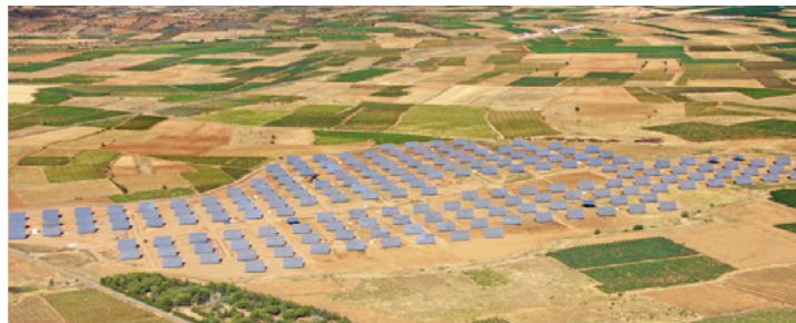
Palacio Cremado 3.15MW Solar Power Plant
