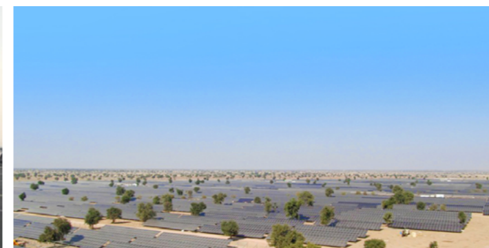
INDIA | Rajasthan 24MW Solar Power Plant
