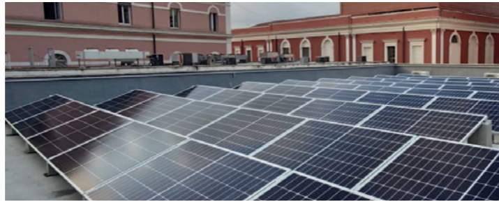
CARTON PACK S.p.a. 2MW Rooftop Solar Plant
