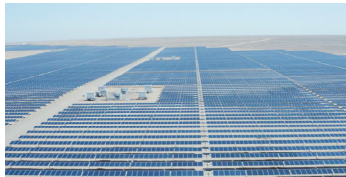
JORDAN | Risha 60MW Solar Power Station
