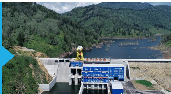
Turgusun HPP-1 25MW hydropower plant
