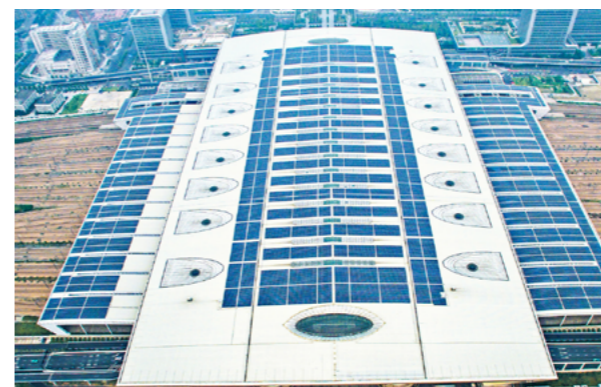
Hangzhou Railway Station 10MW Rooftop Project
