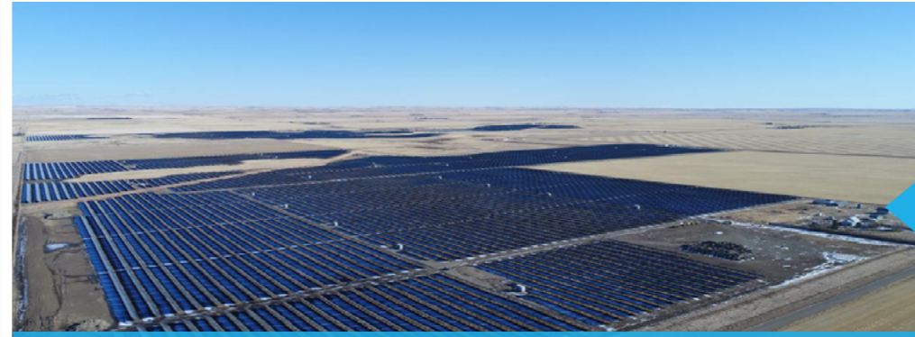
Lo Loma Solar Park Project
